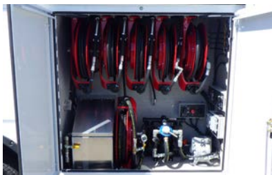
OIL REELS, FILTER DRAIN, WASTE PUMP AND ENPAK CONTROL PANEL
